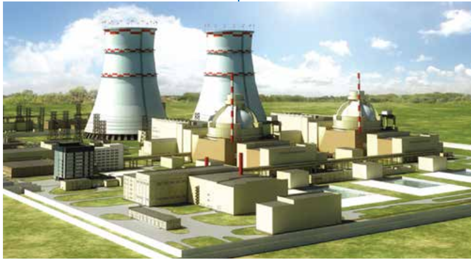
Under construction Rooppur Nuclear Power Plant, Bangladesh.
