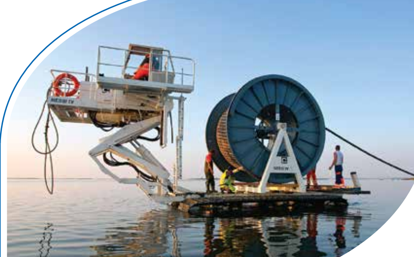
Work of submarine cable in Bangladesh in progress.
